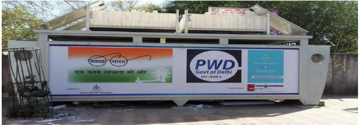
Six Seater Toilet unit developed by PWD at Rani Bagh based on DUAC design.
